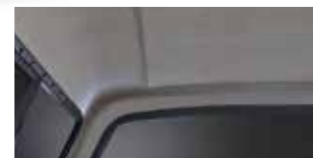
Fiberglass Finish Interior
