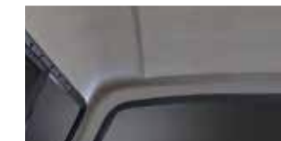
Fiberglass Finish Interior
